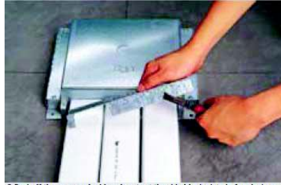
2. Peel off the pre-punched knock-outs at the side blank plate before laying the ductings
