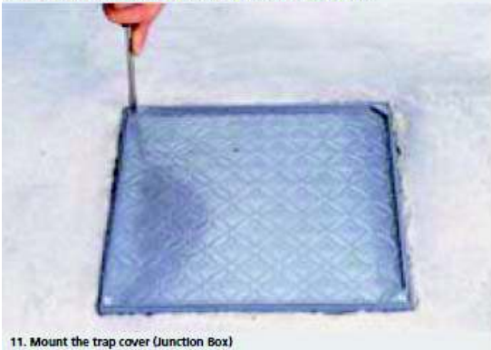
11. Mount the trap cover (Junction Box)
