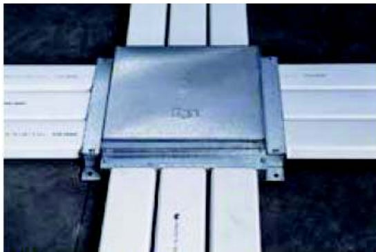
5. The Underfloor Ducting System ready for screeding
