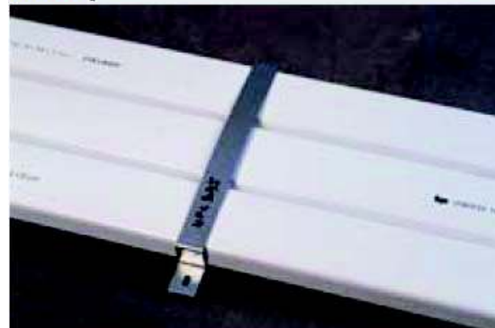
4. Use steel fixing clips to secure the ductings
