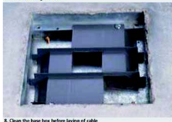
8. Clean the base box before laying of cable
