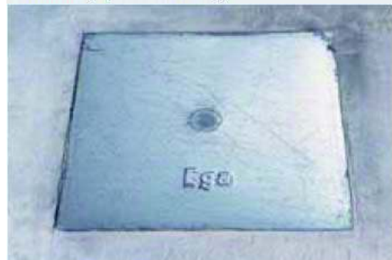
6. After screeding has cured
